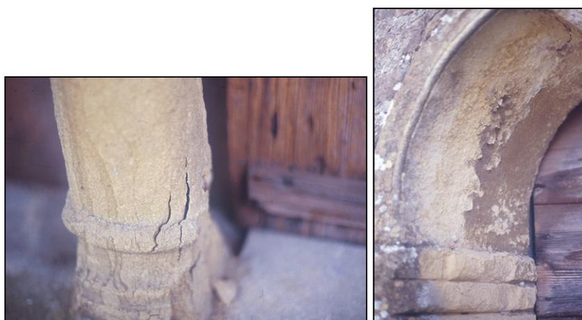
**Fig. 6** Salt crystallization effect on Italian limestone
